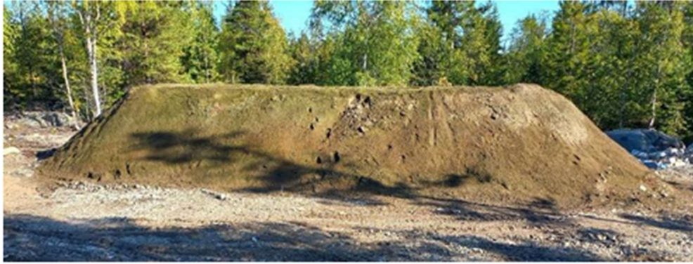
Figure 6: Photograph of pilot scale noise barrier, 3 months after stabilization and solidification (Bjuhr & Andreas, 2023, p. 15)
